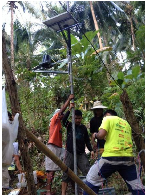
Brgy. Bolodbolod AWS Installation
